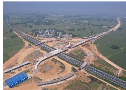
Infrastructure development of the Fangzhao Expressway in Nanyang
