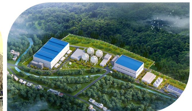
Supported the nation’s first artificially excavated underground compressed air energy storage project
